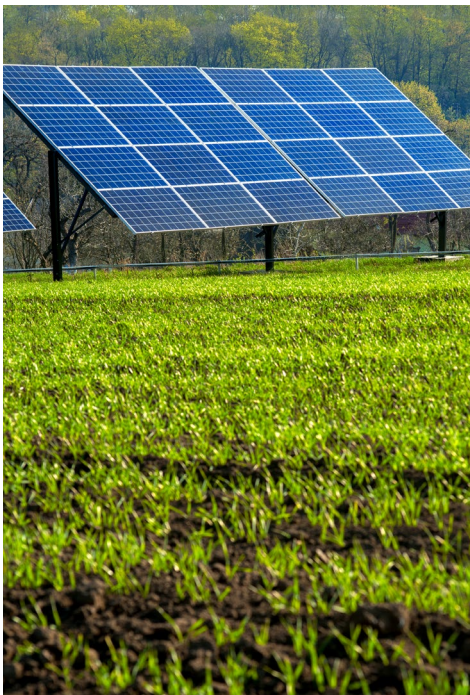
Solar panels are mounted in a field.
